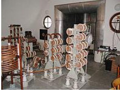
Power ceramic capacitors in a radio-frequency transmitter station
